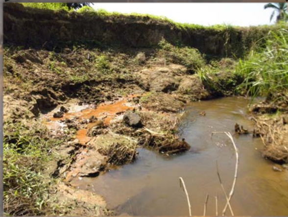
Severe erosion on outside bend of river
