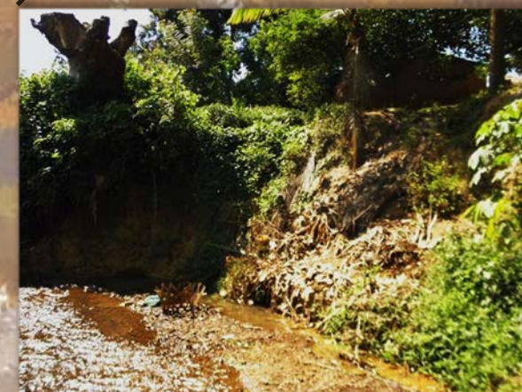
Debris from residential area washing into river
