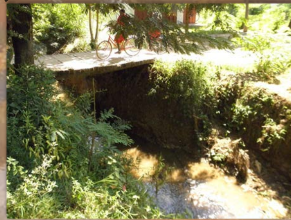
Bridge in Mang'ula B
