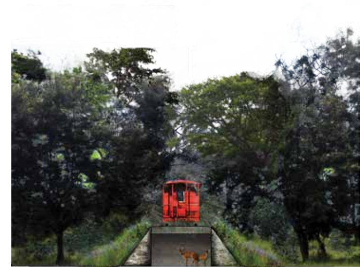
Railroad Animal Movement Culvert
