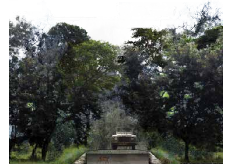
Road Animal Movement Culvert
