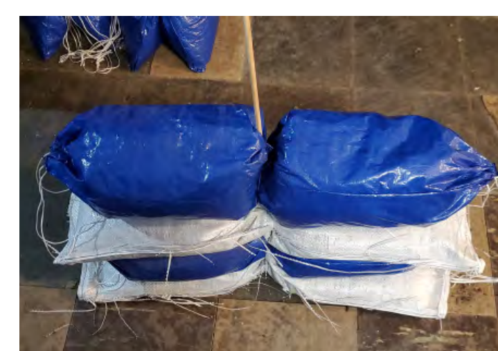
CORNER-STITCH STACK: 2 courses vertically joined with a center dowel
