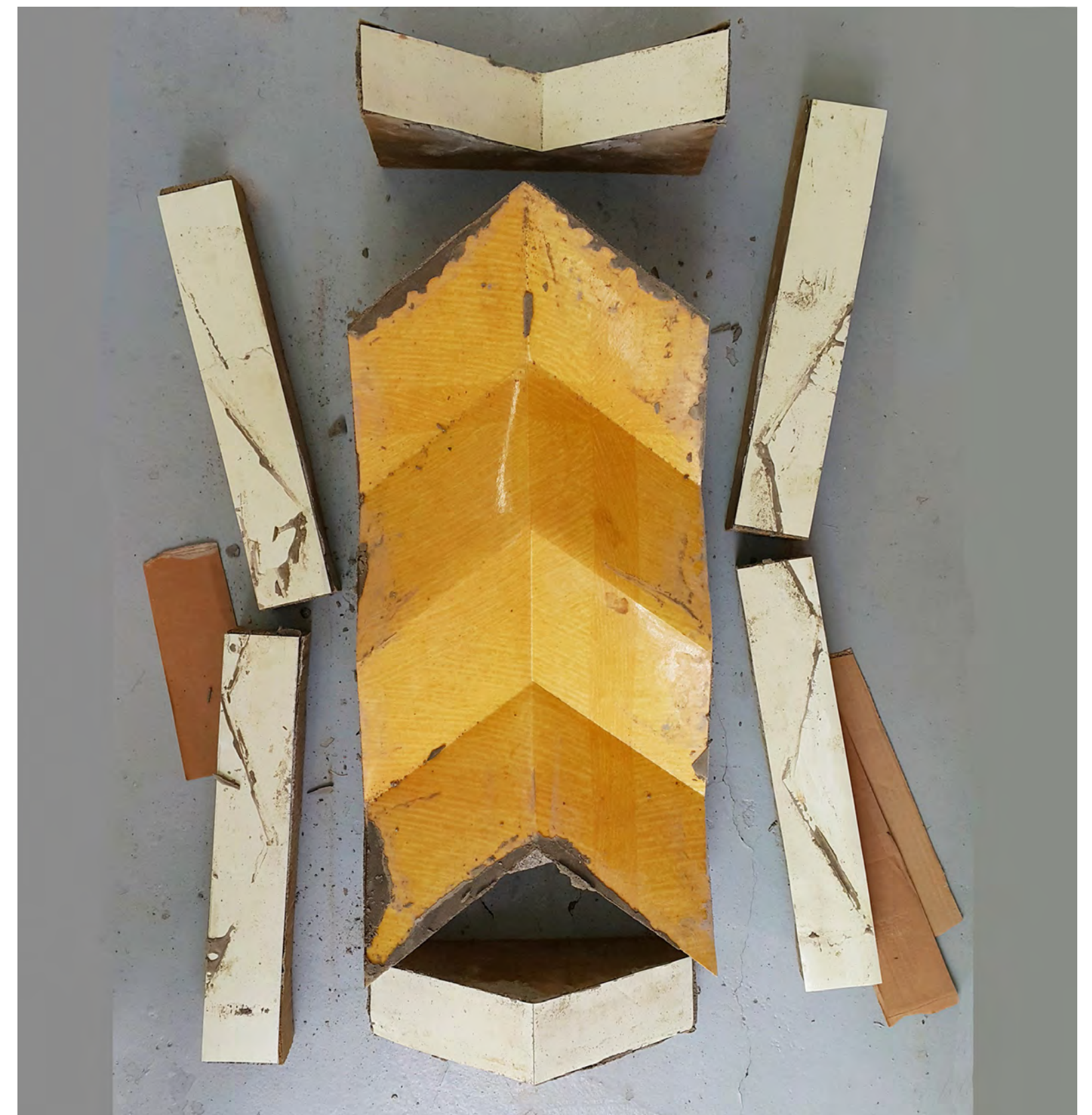
FIGURE 4: THE FORMWORK CAN BE REUSED SEVERAL TIMES THANKS TO THE KOREAN VINYL (OBTAINED FROM WASTE FLOORING VINYL). THE FORMWORK KEEPS ITS QUALITY FOR REUSE. PHOTO: M. SHAFFER
