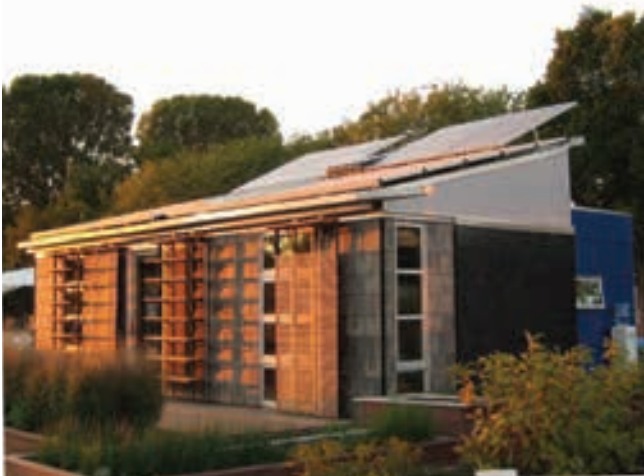
Fig. 1: MorningStar PA as exhibited at the Solar Decathlon on the National Mall in Washington D.C. in October of 2007. (Courtesy of the 2007 Penn State Solar Decathlon Team and the Center for Sustainability at Penn State)
