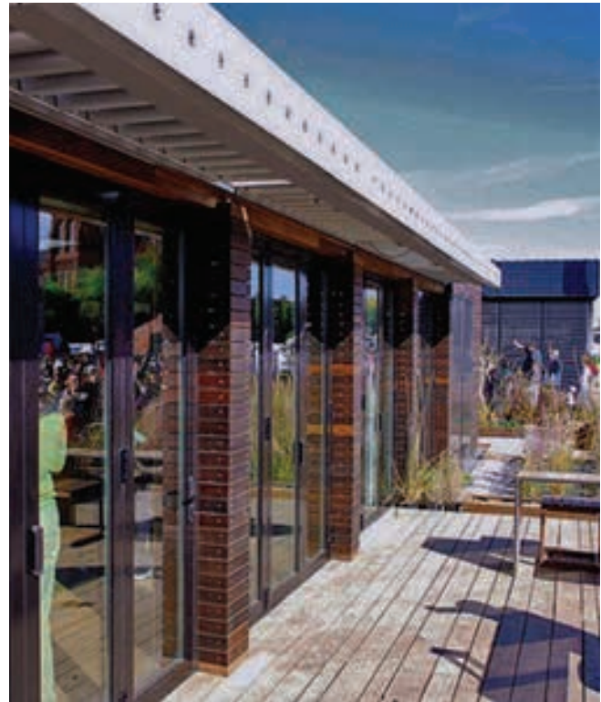
This solar-electric shading canopy tracks the sun
