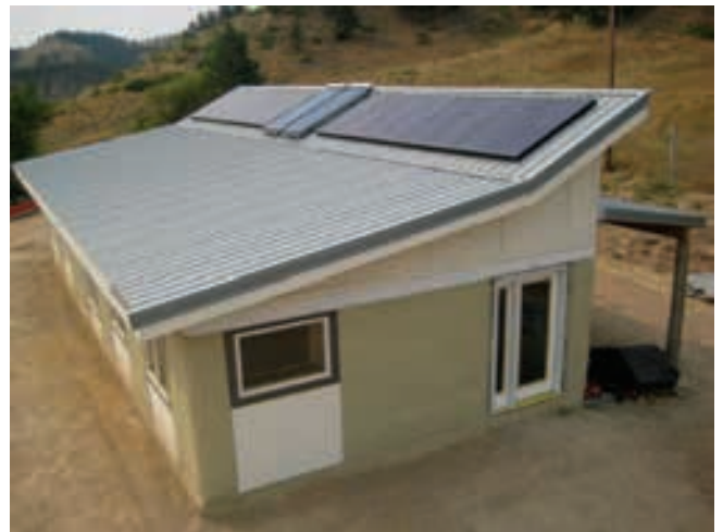
Fig. 2: American Indian Housing Initiative’s MorningStar MT. (Courtesy of the 2007 Penn State Solar Decathlon Team and the Center for Sustainability at Penn State)
