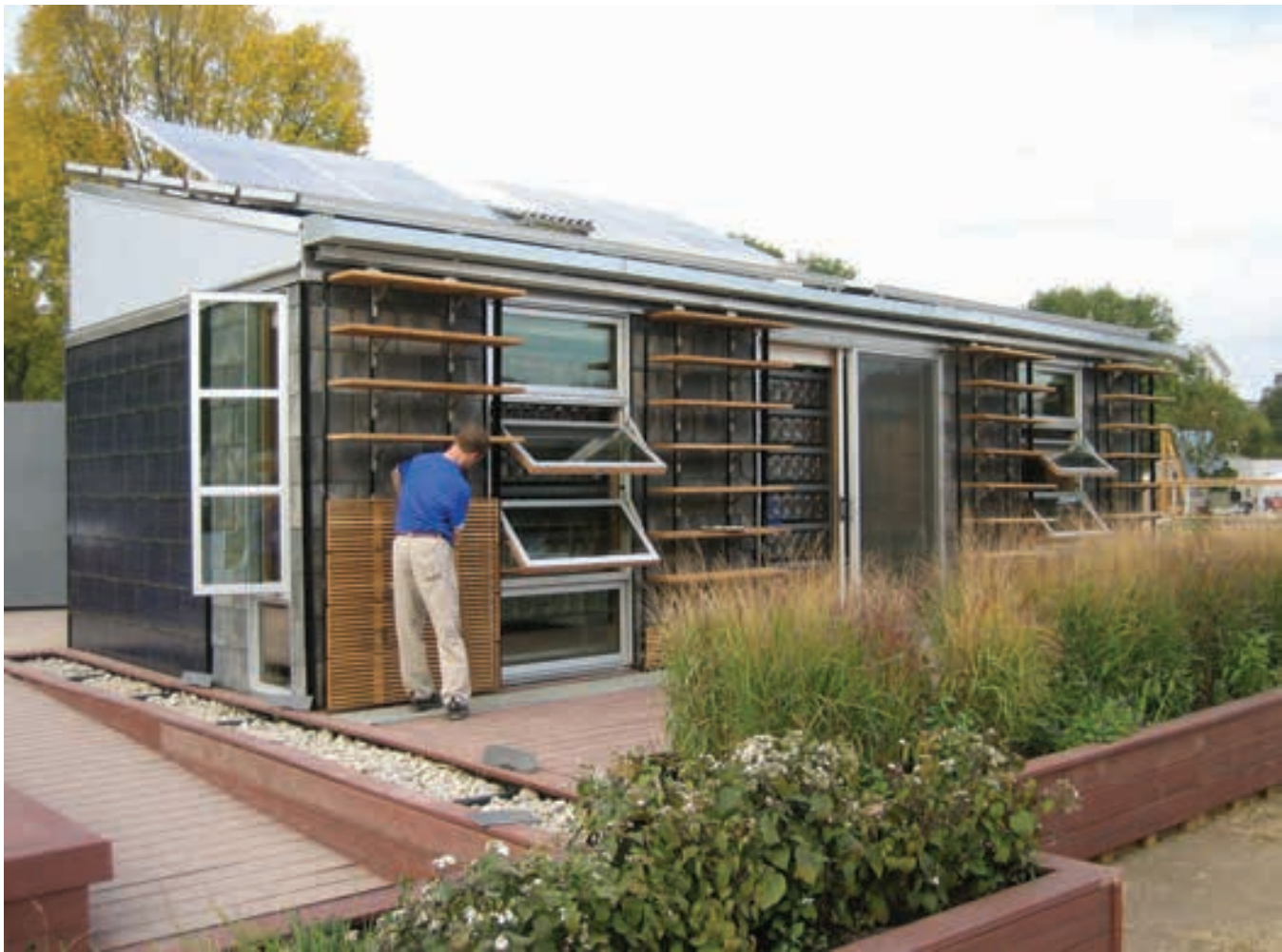
above: solar slate panels are a modern play on the reclaimed slate cladding material.
