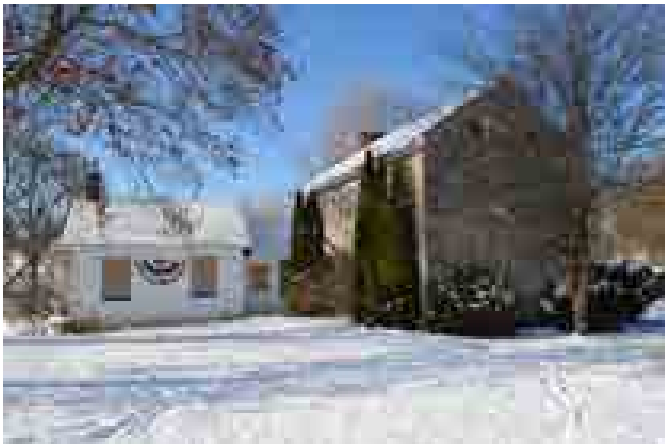
Rear of farmhouse with attached "summer kitchen"
