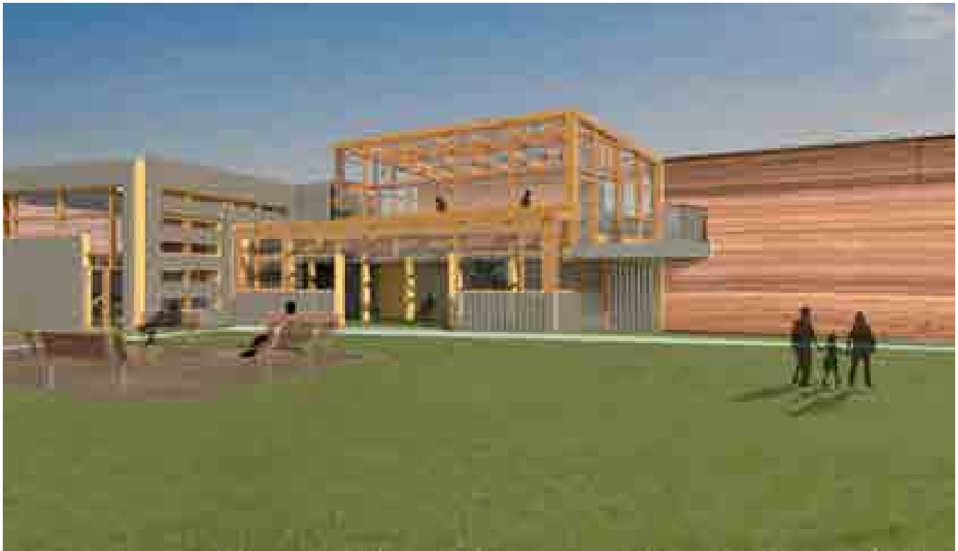
Welcoming view indicating rammed earth wall from CLT walls and wooden mullions.
