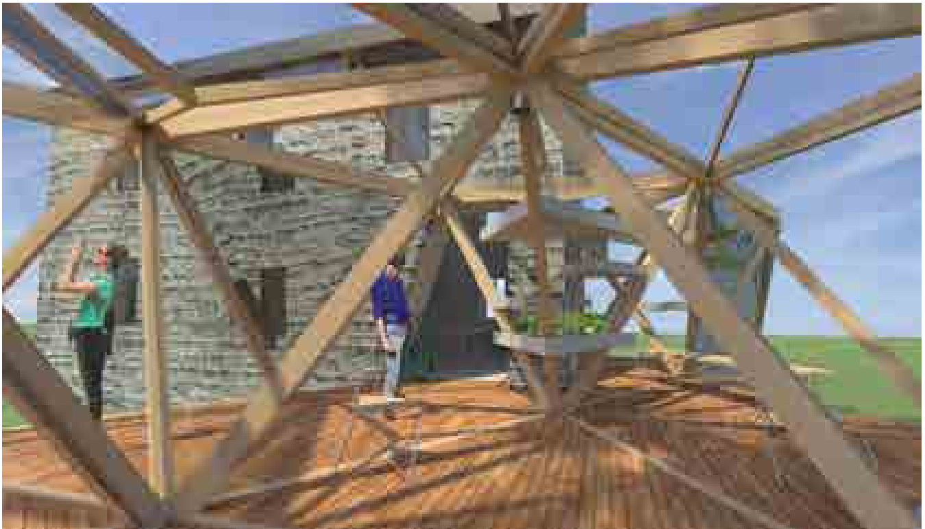
Addition Interior New addition space made of light weight modular construction system.
